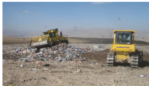
On this picture you see on the right a caterpillar covering the cell with soil and on the left hand a special compactor.
